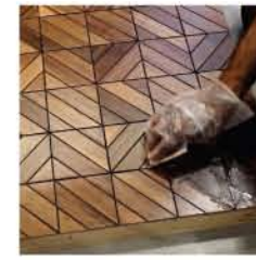
Step-9: Fill epoxy grout material
