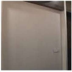
Step-1: Provide a dry & levelled wall surface
