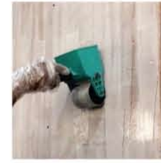
Step-4: Apply glue to liner material
