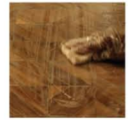
Step-10: Clean excess grout from wood surface
