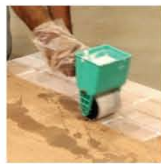
Step-3: Apply glue to liner material on floor
